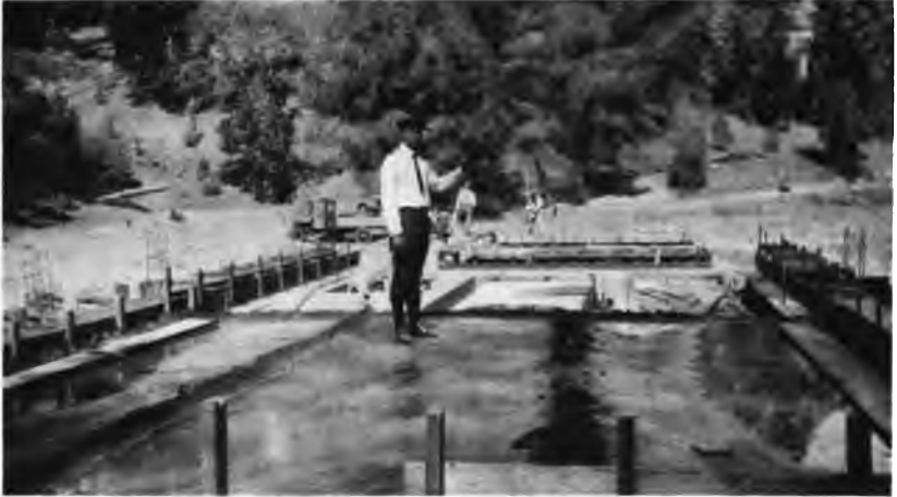
Engineer J. B. Woodson of Division VI inspecting bridge work.
